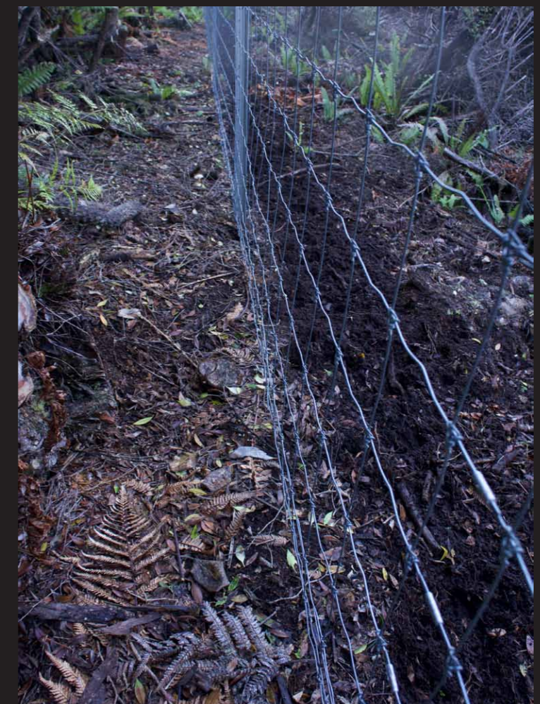
The fence from coast to coast to the north of the Spit/Old Neck now provides a boundary for deer control operations. Note the deer tracking outside the fence from animals trying to enter. Vigilance will always be required as some deer may still swim to The Neck.
