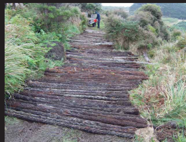
'Corduoy' laid laterally to enable water flow
